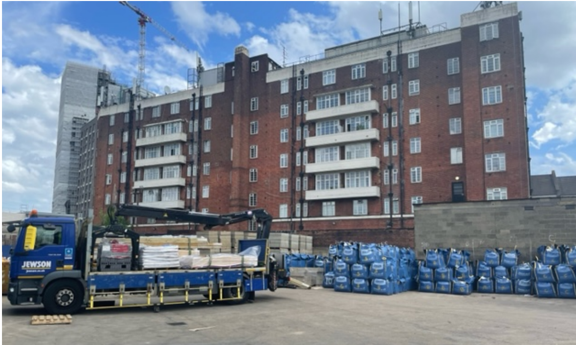
Figure 16: Rear Elevation of Acton House
