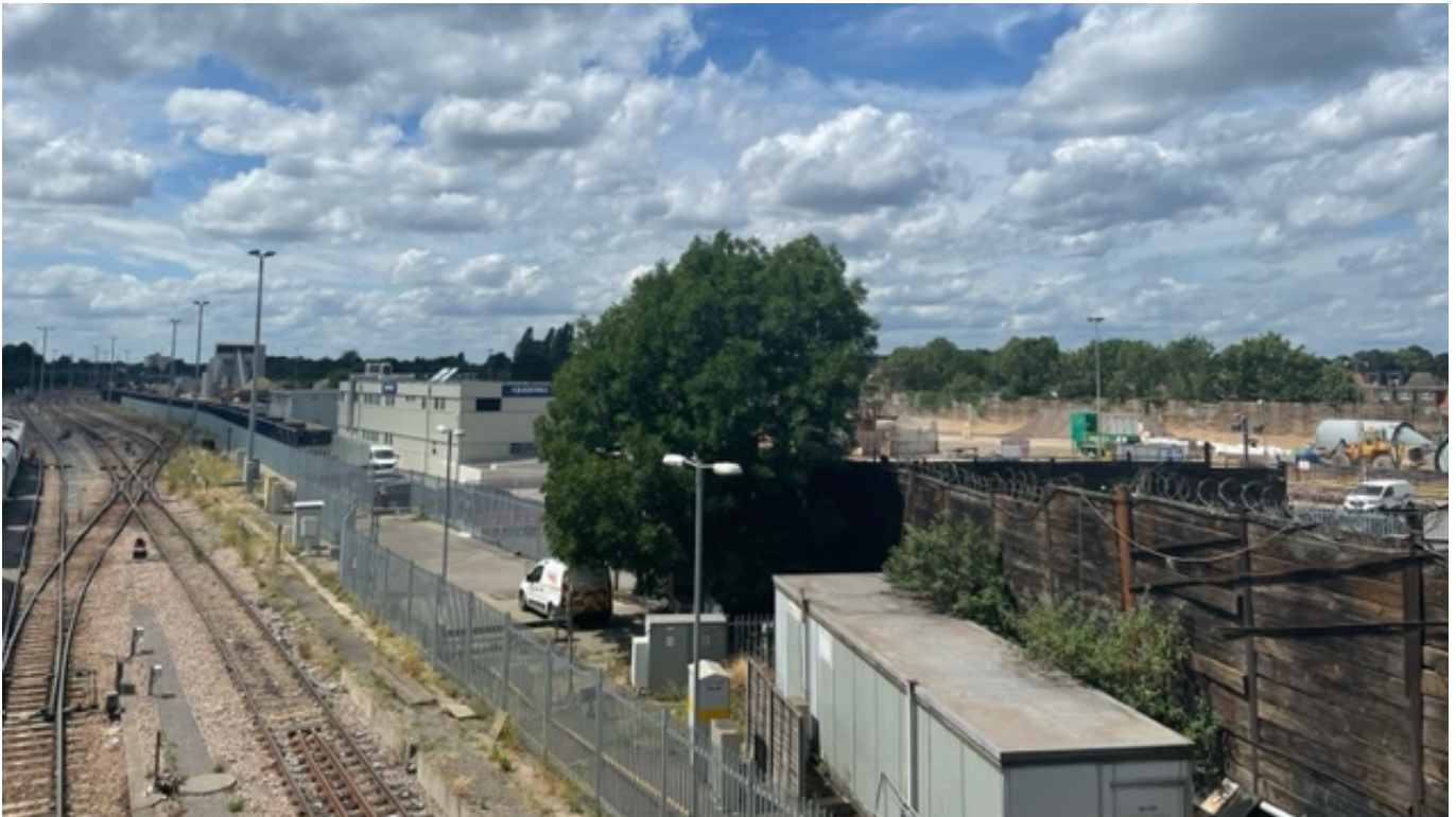
Figure 2: Industrial activities on northern side of railway
