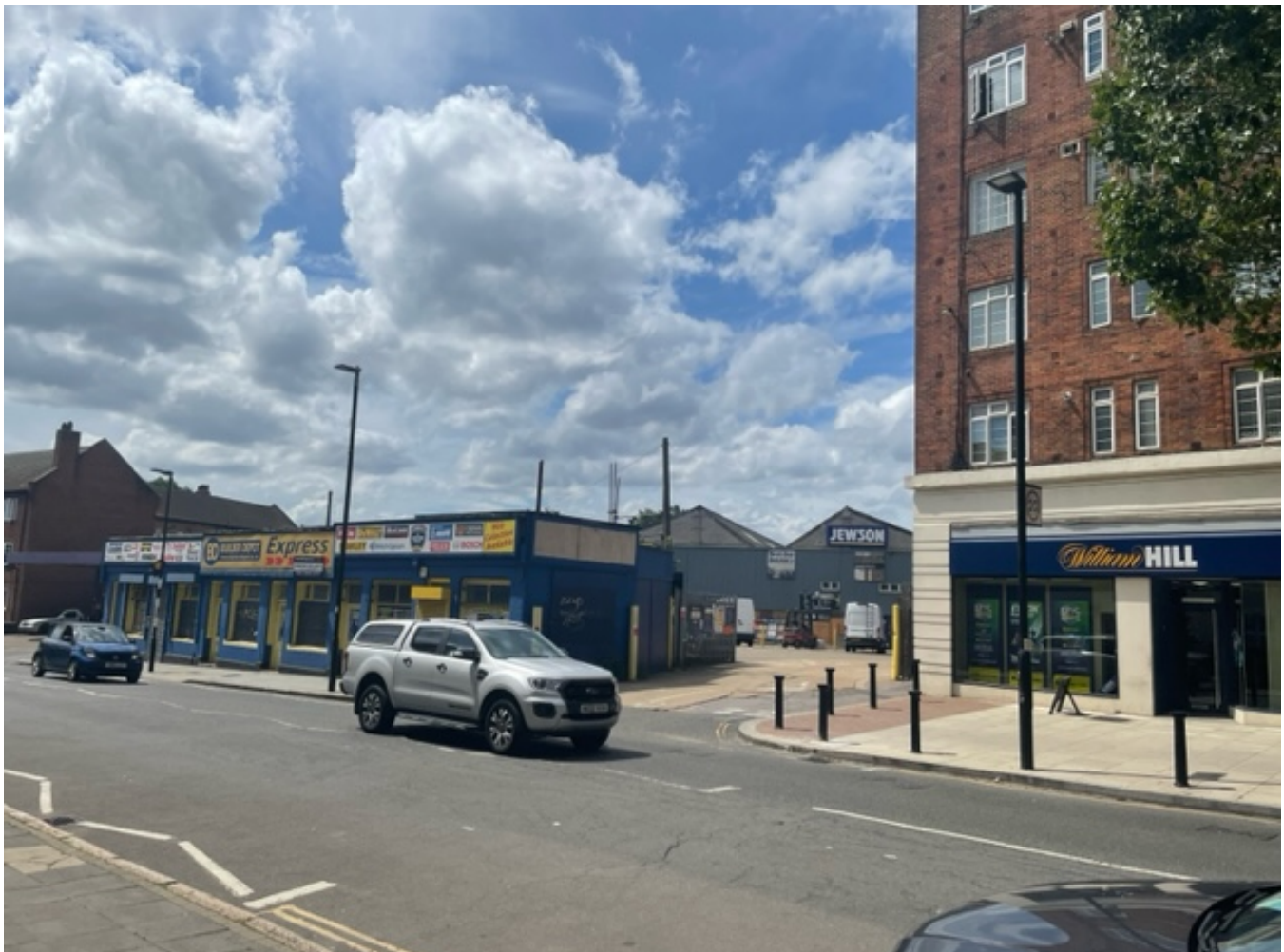
Figure 1: Frontage of Site showing crossover, Acton House and shopfronts to be demolished.
