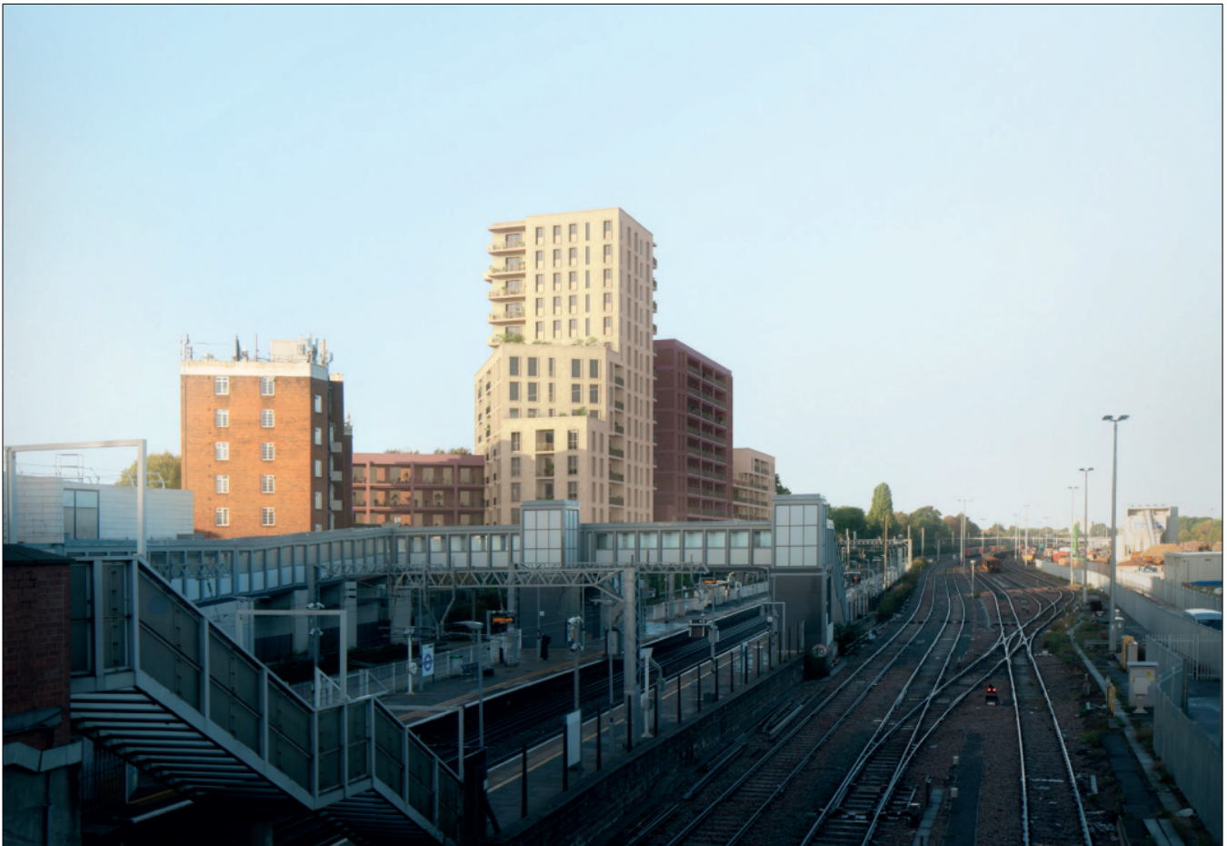
Figure 15: View from Acton Main Line Bridge
